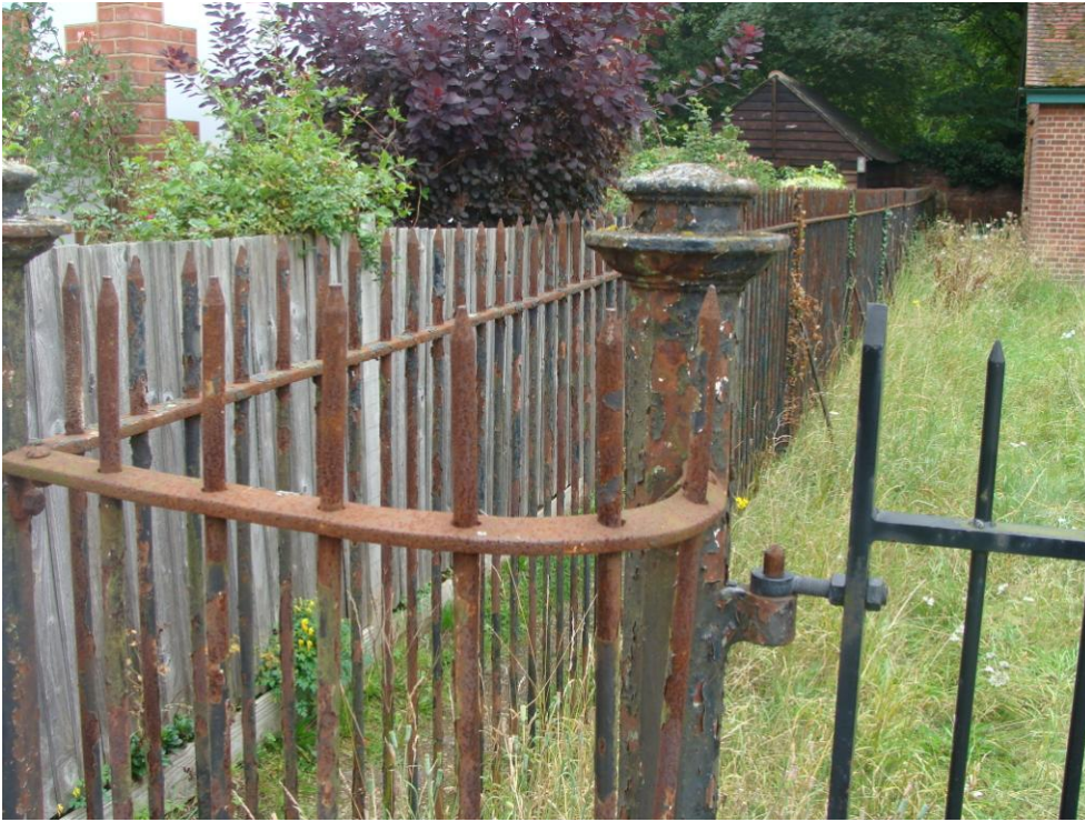
Picture 16 – Metal fence to side of Thames Water facility, worthy of retention and in need of repainting.
